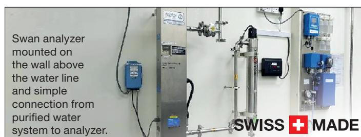
Swan analyzer mounted on the wall above the water line and simple connection from purified water system to analyzer.
